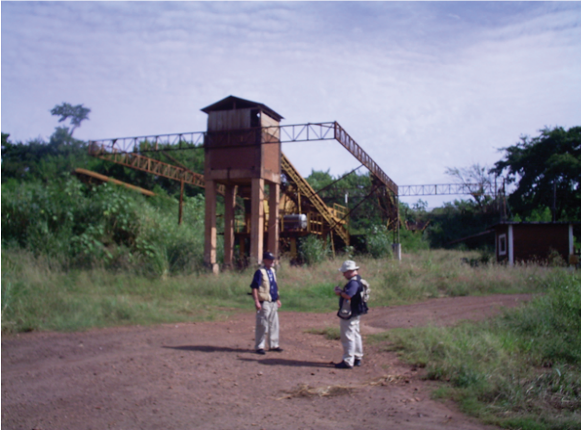
View of the former processing plat for the calcite with 3%-5% phosphate for the local farmers.
