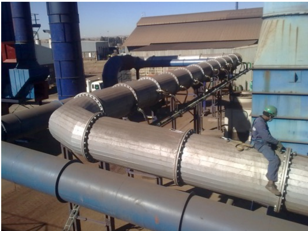
2 x Fume extraction with energy recovery
