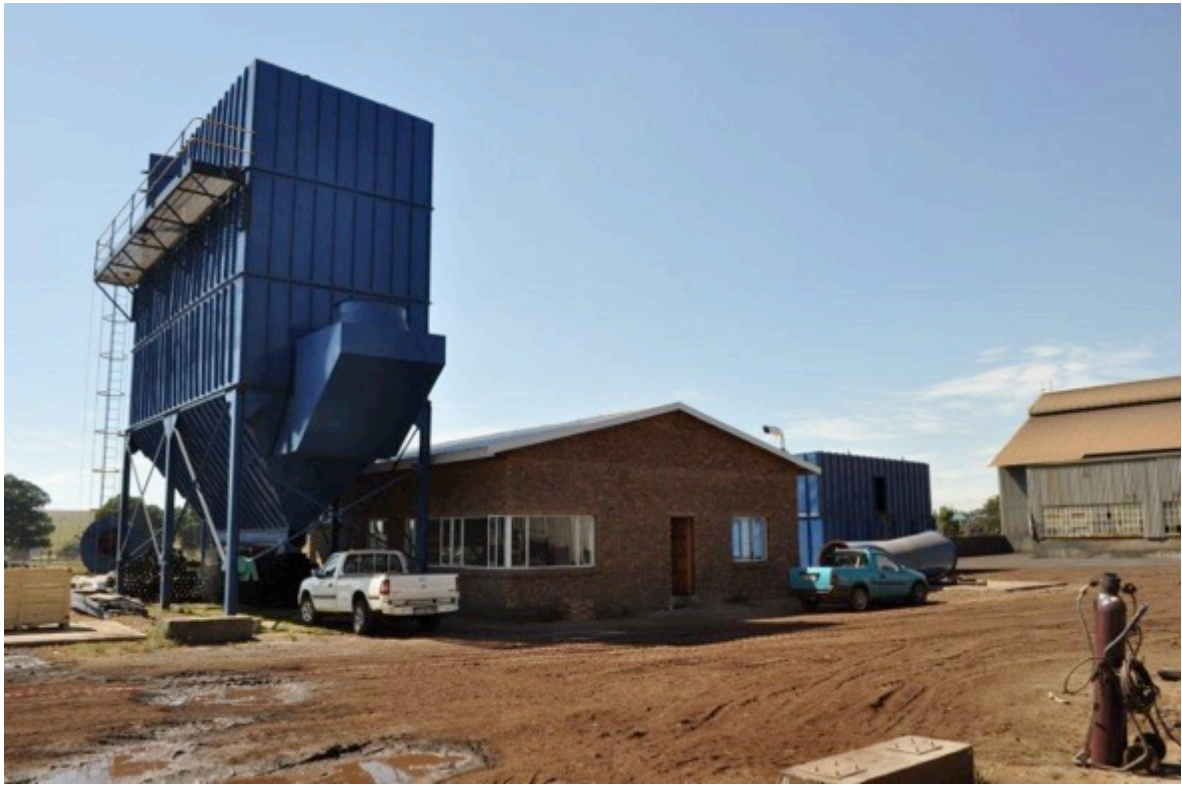
Bag filter 1 erection
